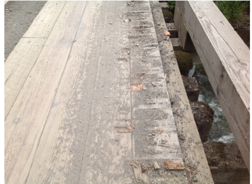
tracked machine recently walked over
