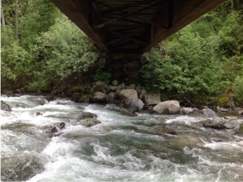
Left Bank Abutment when facing downstream
