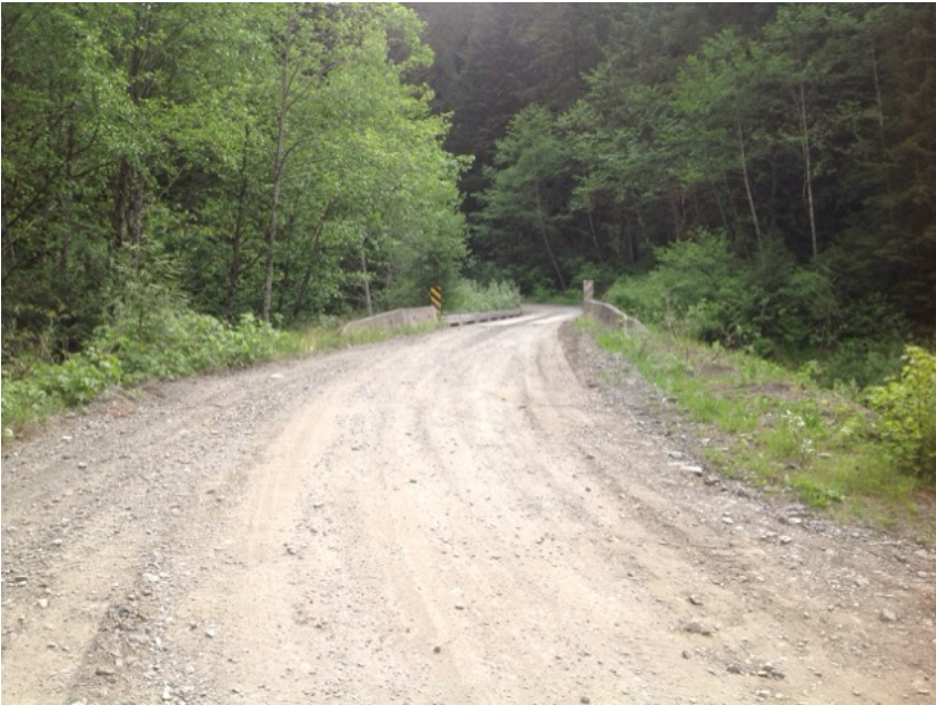
Approach from Right Bank when facing downstream
