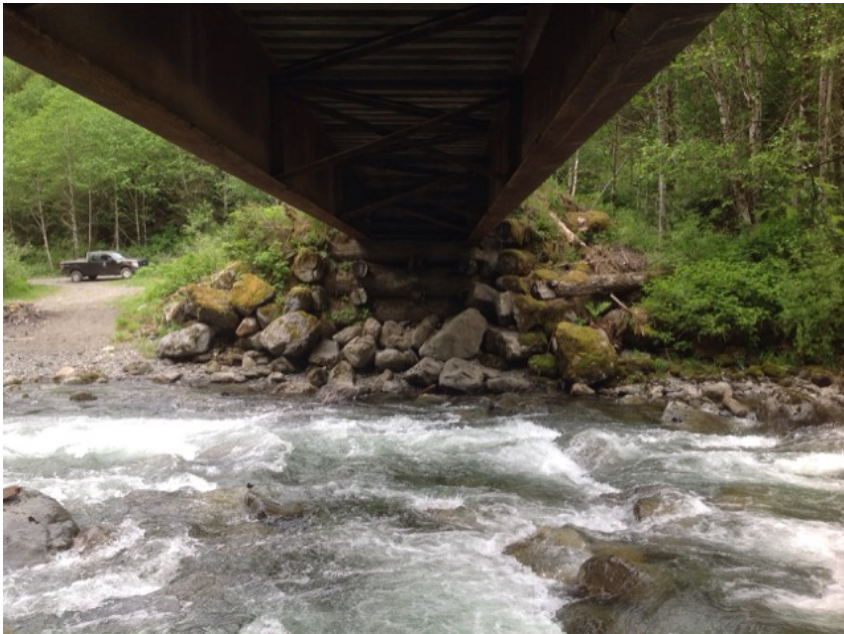
Right Bank Abutment when facing downstream
